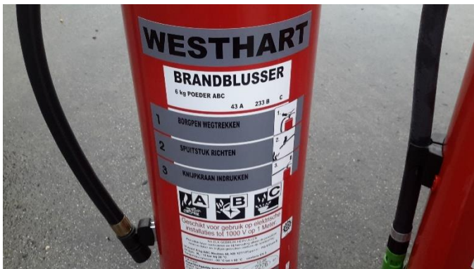
Standard EN3-7 certified powder unit (6 KG)
