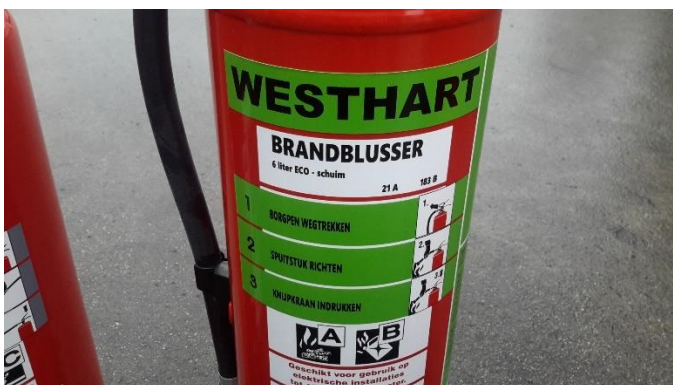
Standard EN3-7 certified foam unit (6 L)
